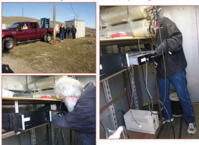
At the Repeater Shack and Installing the Repeater
